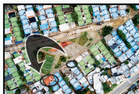
An aerial view of where we are currently and where the new building will be. It's a great location! The government just finished renovating this park.
